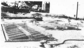
Fig. 1—Prototype solar stills at the Experiment Station in Syros.
